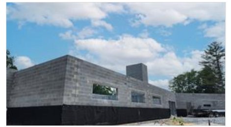
New Connestee Falls Fitness Center, completion expected mid 2024
